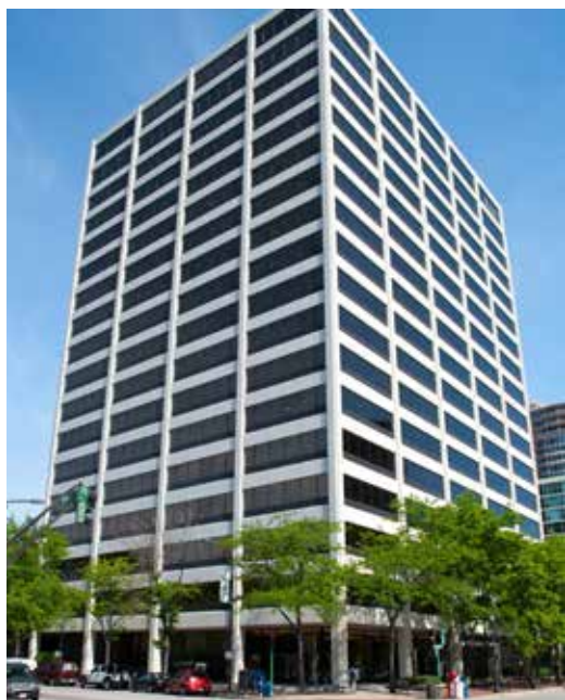
One Rotary Center (ORC) in Evanston, Illinois, USA.
